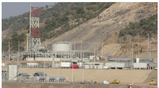
Intermediate pigging and pressure reduction station
