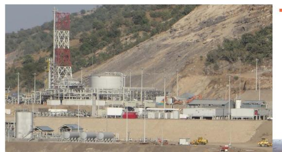
Intermediate pigging and pressure reduction station
